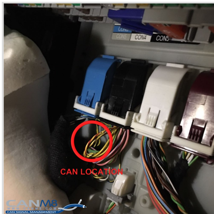
CAN Bus Wiring
